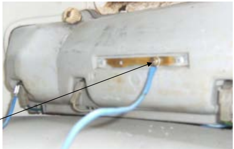
Self tapping screw to earthing strip
